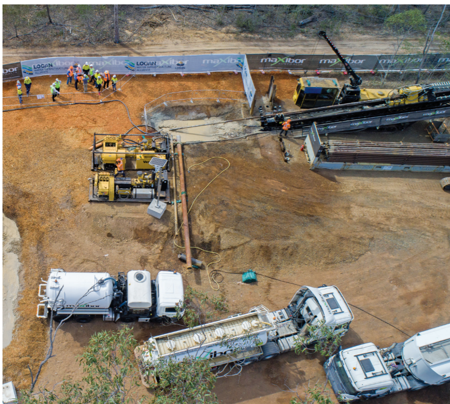
Maxibor was responsible for the HDD installation of the polyethylene high stress crack resistant pipe, supplied by Iplex.
